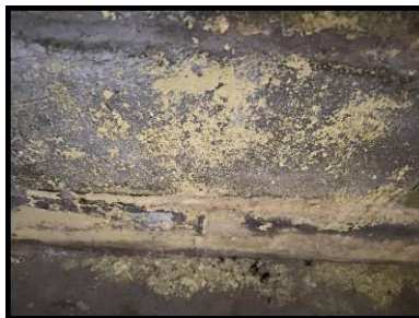
Efflorescence on Foundation Wall
